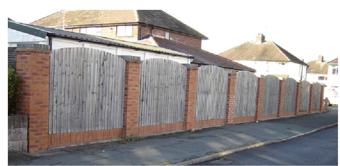
WALL WITH FENCE ABOVE
