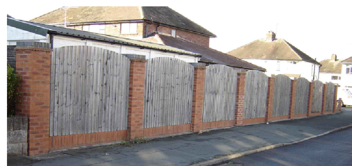
WALL WITH FENCE ABOVE
